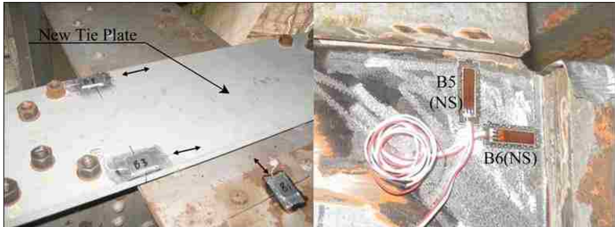
Figure 2-9: Strain gages installed on the tie plate (B3, B4), on the top flange of the girder (B1) and on the cantilever bracket web (B5, B6)
