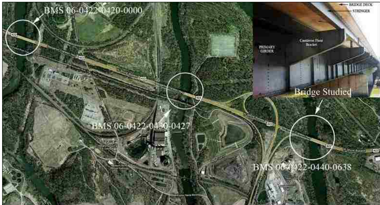
Figure 2-1: Bridge location (Google Maps 2010) and view of bridge looking east from Abutment 1
